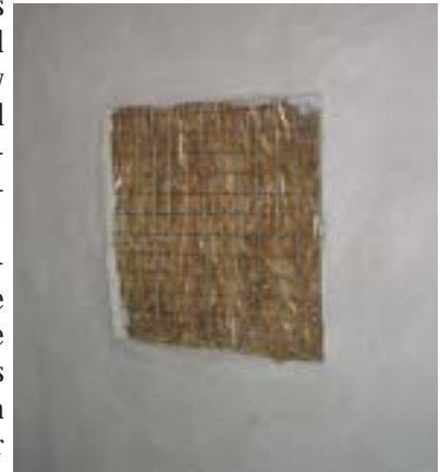
The "Truth Window" is a common feature of modern day straw bale construction, proving to visitors what's inside the concrete stucco!
